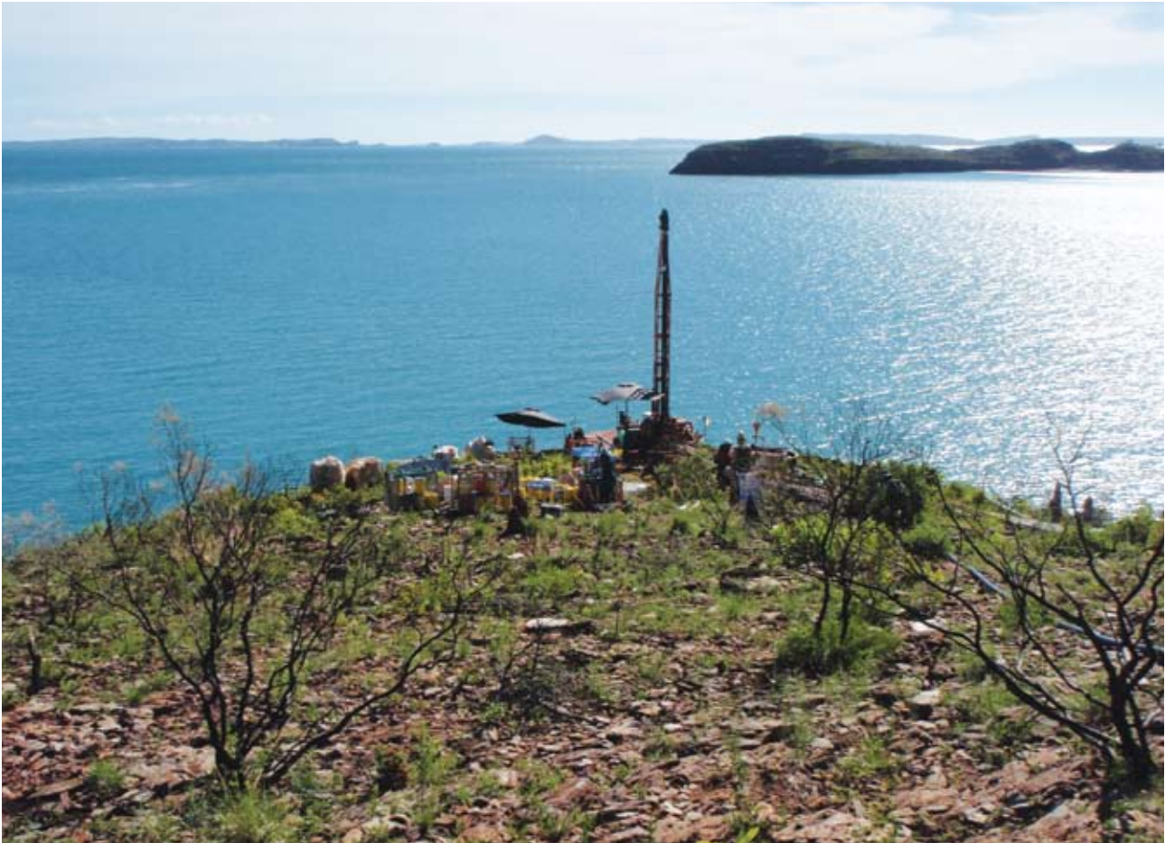
Drilling operations on Hardstaff Peninsula, Irvine Island.
