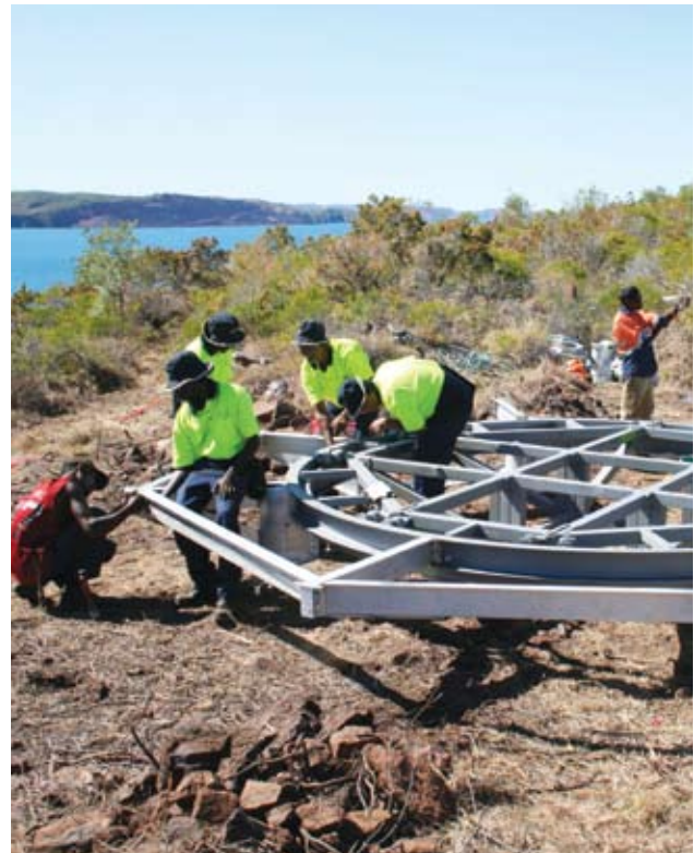
Mayala employees constructing the UDP on Hardstaff peninsula prior to drilling.
