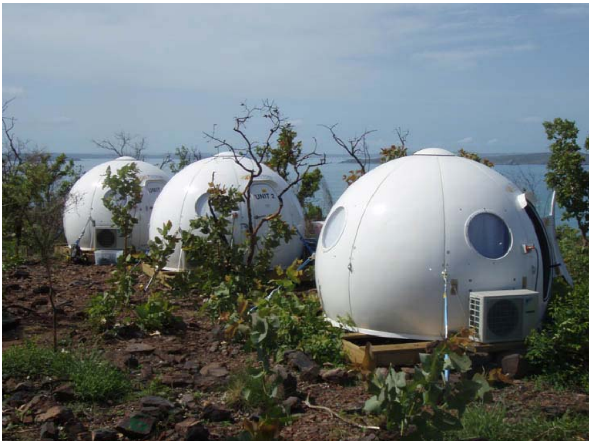
Figure1. Accommodation pods on Irvine Island. The pods can be easily moved and are designed to cope with extreme climatic conditions.
